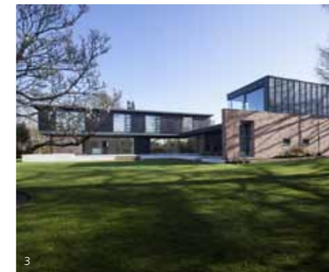
Front, 1 Stormy Castle, Llanmadog (photographs: Charles Hosea) 2 Westra Nook, Dinas Powys (photograph: Charles Hosea) 3 Millbrook House, Lisvane, Cardiff (photograph: Ståle Eriksen) 4 Llandegfedd visitor centre and watersports centre (photograph: Jonathan Vining) 5 The Towns of Wales , second edition, dust jacket (University of Wales Press) 6 Coriolanus , Hangar 858, MoD St Athan, Vale of Glamorgan, August 2012 (photograph: Jonathan Vining)
