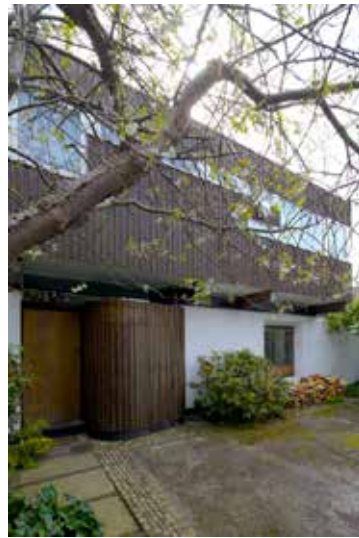
Previous pages: sunlight is reflected from the pool on to the ceiling of the south-facing living-room. Above, the front door and cloakroom pod. Right, the timber-clad first floor cantilevers over the masonry and glass walls below on four glulam beams
